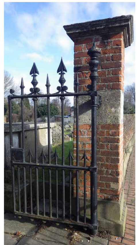
Figure 29: Gate and brick wall to churchyard.
