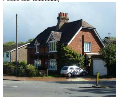
Fig. 36: Former Post Office
